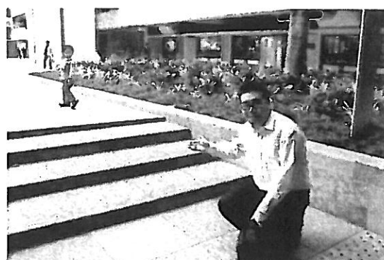
(E) 樓梯需加設燈槽
